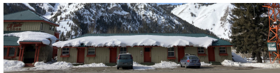
Lift Tower Lodge Blaine County Housing Authority-owned
